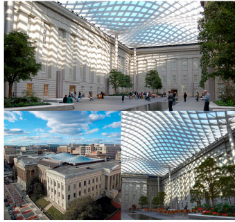
Smithsonian American Art Museum - Washington, DC 2016 Vulnerable horizontal glass can become easily corroded and quite labor intensive to clean. Invisible Shield coating was applied many years ago to preserve the glass and reduce the cleaning overall.
