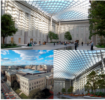
Smithsonian American Art Museum - Washington, DC 2016 Vulnerable horizontal glass can become easily corroded and quite labor intensive to clean. Invisible Shield coating was applied many years ago to preserve the glass and reduce the cleaning overall.
